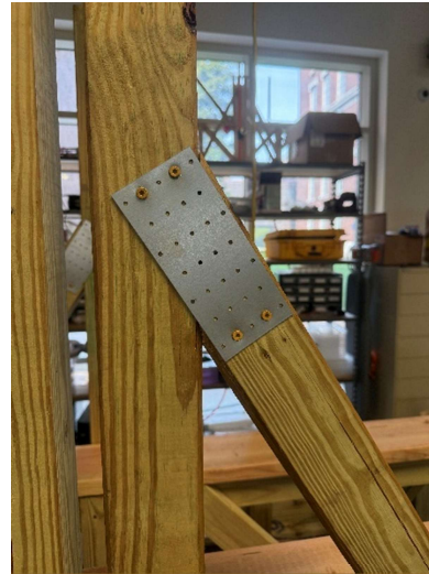
Figure 18: Chute with its support connected by a piece of metal sheet.
